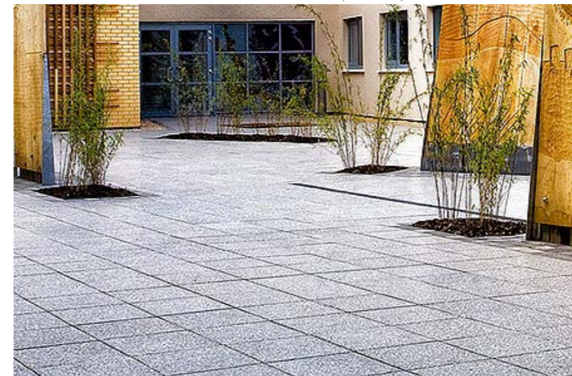
Pre-cast concrete paviours to residential terraces and podium garden
