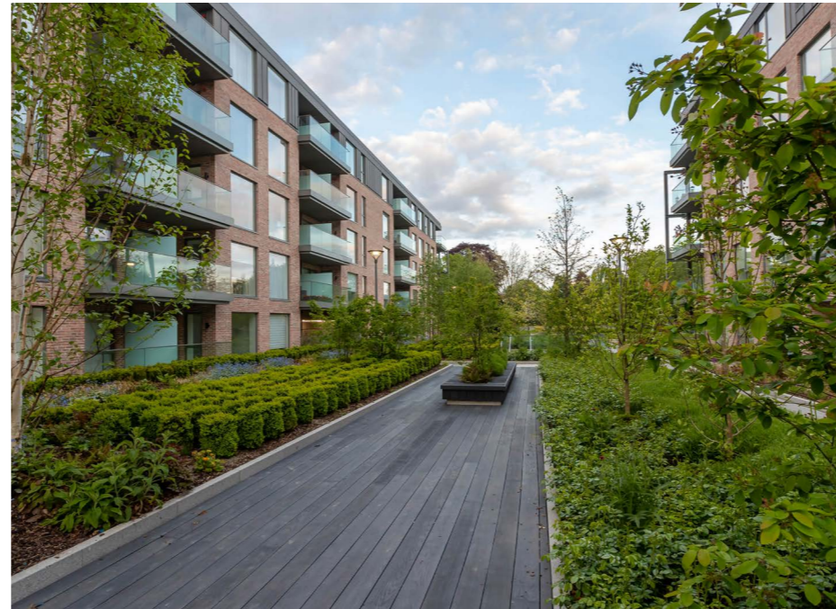
Over podium courtyard planting: Planting soil depths achieved for tree planting over podium deck through localised mounding.
