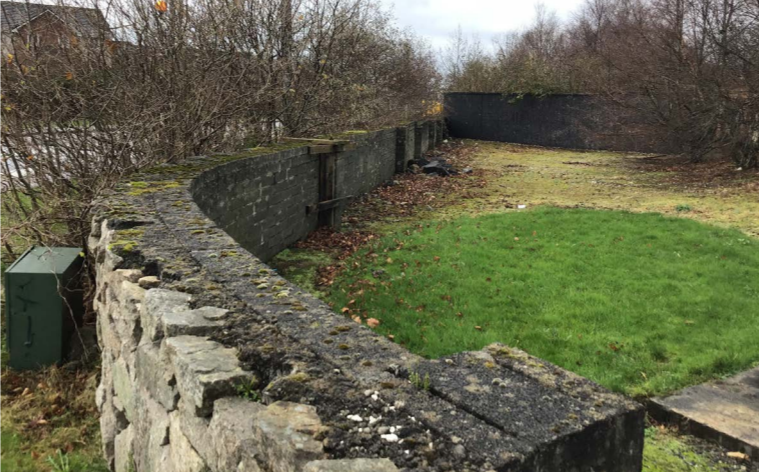
Existing stone faced blockwork wall along Gort Ná Bro/ Western Distributor Roads
