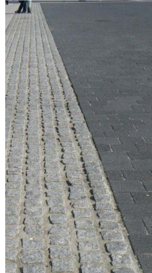
Natural stone setts to public realm/ private thresholds
