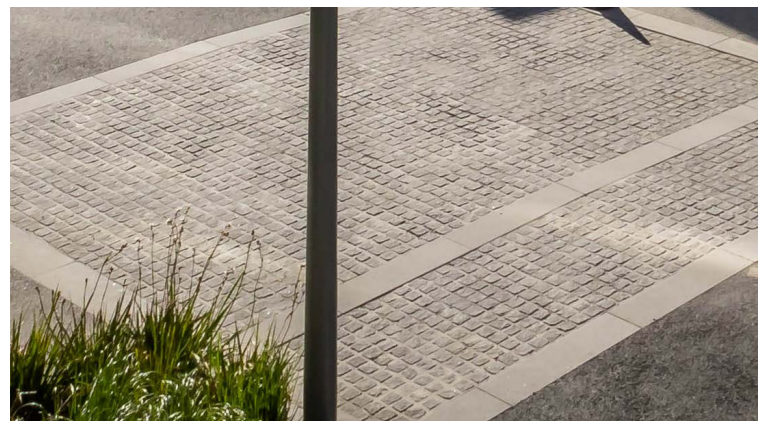
Raised table crossing - Pedestrian priority & traffic calming
