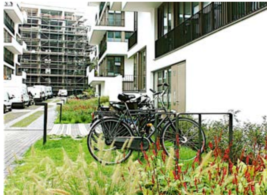
Ground floor residential with defensible space garden planting
